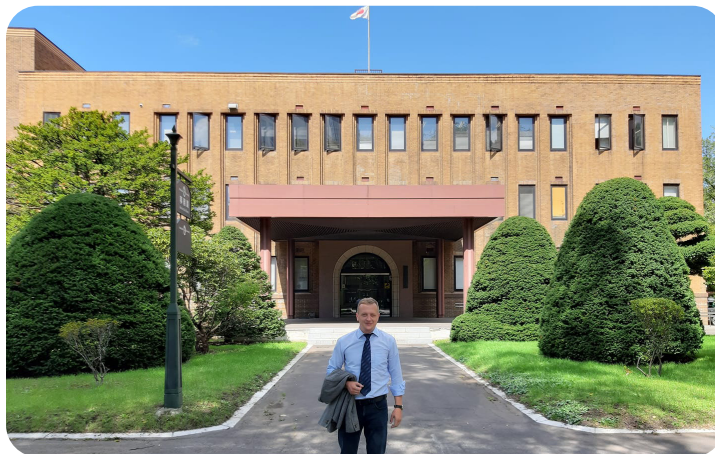
In front of the main administration building of the University
